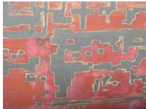
Square blast cleaning
