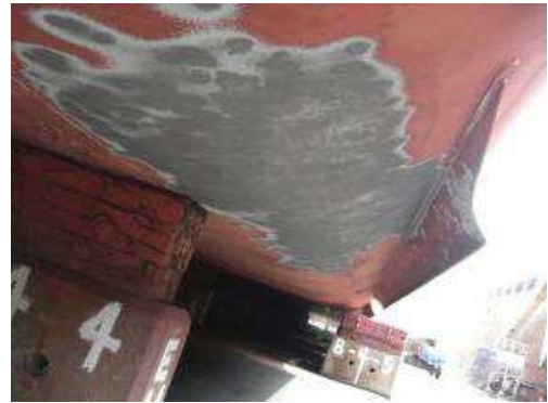
Rust scale or blistering (Partial blast cleaning)
