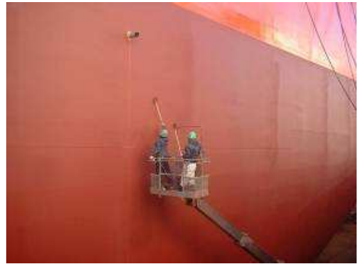
Removal of paint dust before final coating
