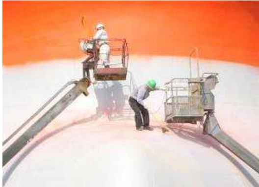
Removal of paint dust of finish coating adhered on bulbous bow
